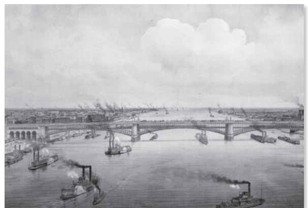
Figure 2.6 St. Louis Eads Bridge
